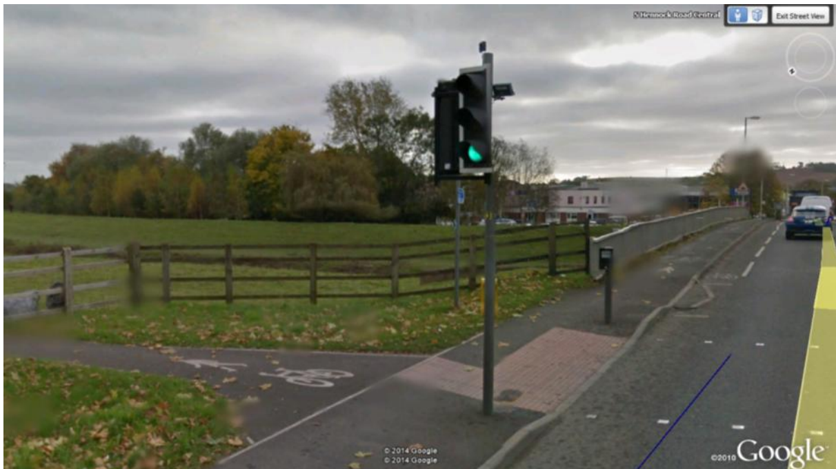
Figure 6-6: Road bridge over drainage channel on Hennock Road Central
